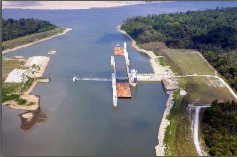
Photograph: Montgomery Point Lock and Dam at the confluence of the White and Mississippi Rivers
